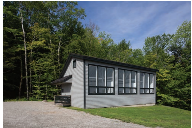
HELEN FRANKENTHALER STUDIO by Neil Kittredge, Beyer Blinder Belle COMPLETED 2019
