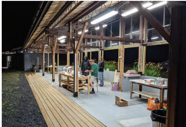
MOFFETT/GOBER SCULPTURE PAVILION by Neil Kittredge, Beyer Blinder Belle COMPLETED 2019
